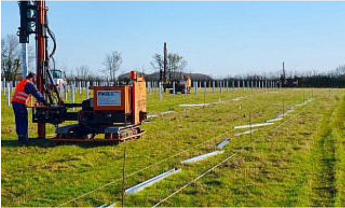
Ramming of the support profiles.
