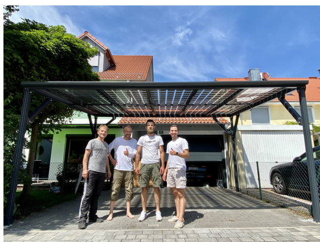
Carport special construction (2,5 kWp)
