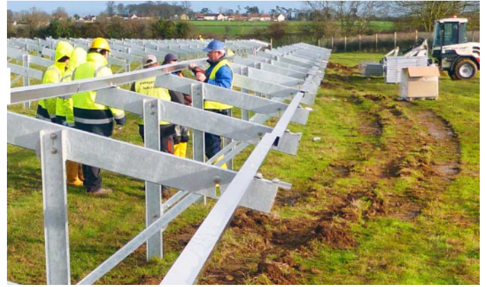
Mounting of the project-specific substructure on the pole foundations.
