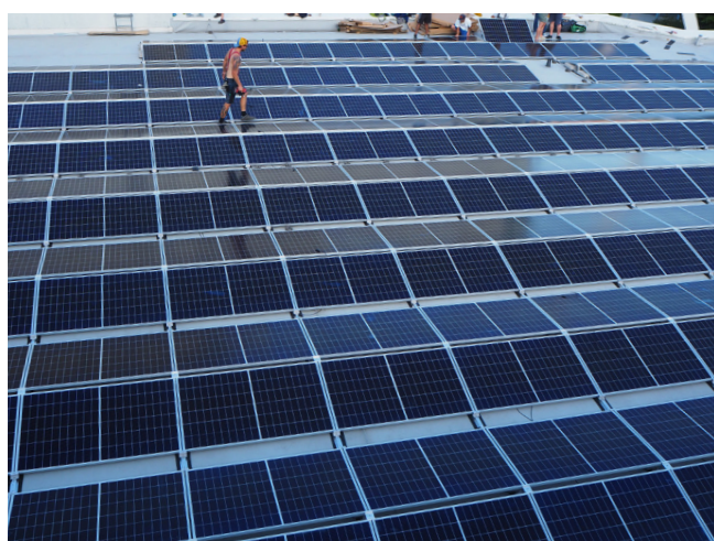
PV roof installation with HC Modules (712 kWp)
