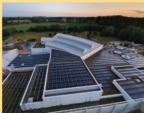
Large PV Installations (p. 43)
